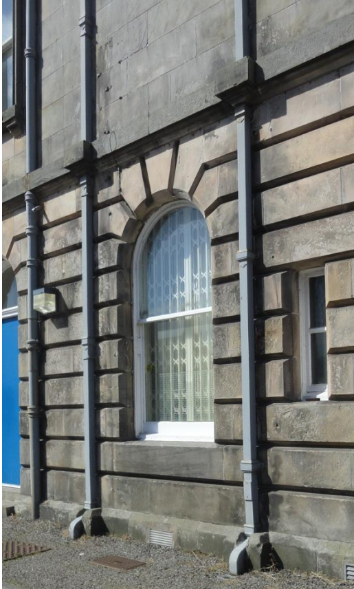
Figure 22. East elevation (1862), channelled masonry, square section downpipes.
