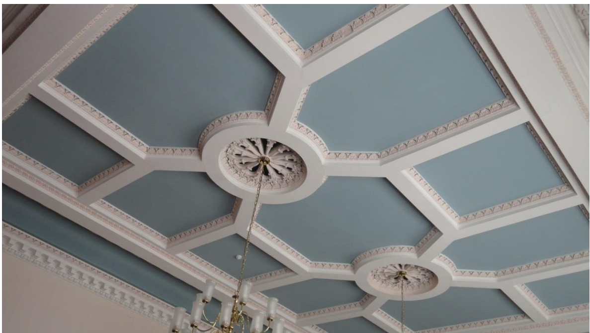
Figure 32. Decorative plaster ceiling of Court Room, as per Campbell Walker's plan.
