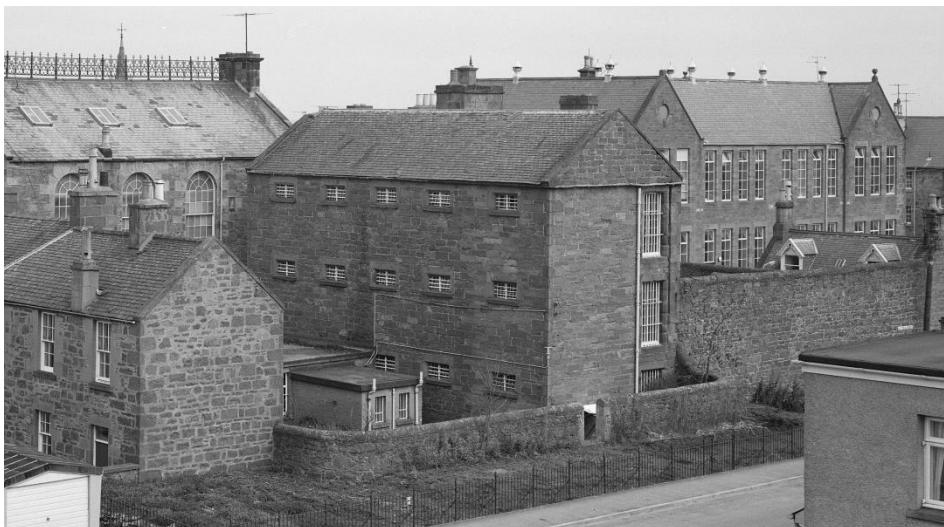
Figure 9. The 3-storey, 4-bay prison cell block added 1842 and lock-up and apartment of 1847. Photograph taken 1983, showing further contextual changes and an additional bay to the south east, prior to their demolition in 1983. © Courtesy of Historic Environment Scotland.
