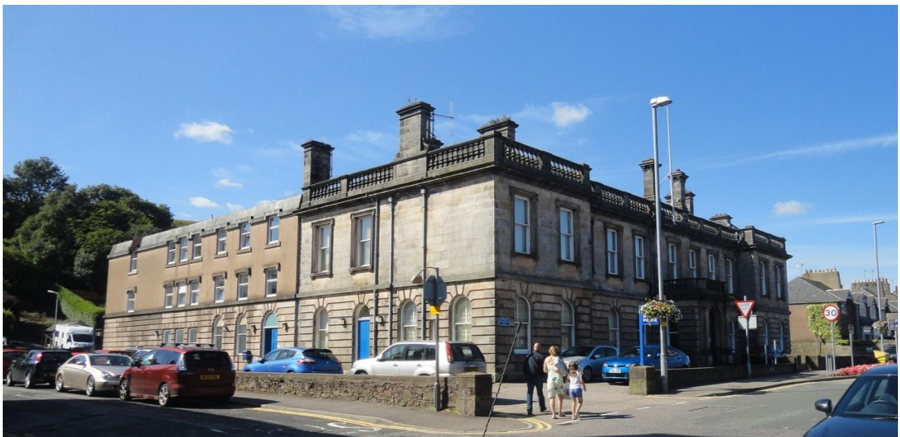
Figure 23. Stonehaven Court Building from the north-east showing contrast of 1983 extension to the south east (left).
